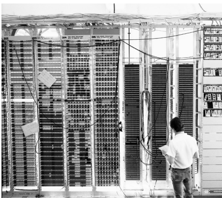
Jack-field and Cross-Connect
